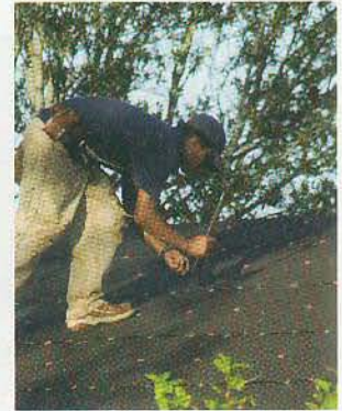
▲ fix the roof
