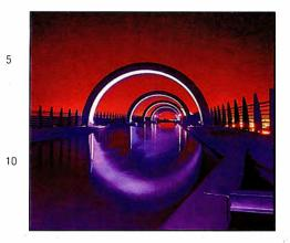
*Falkirk Wheel* (Falkirk, Scotland, 2001) The Falkirk Wheel is the world's only **rotating** boat lift. Its steel arms each hold a water-filled tank into which boats can sail. As the wheel rotates, so do the arms, raising and lowering the boats a distance of 25 meters. The wheel is very energy **efficient**, using about two kilowatt-hours to make a full rotation. That's about the same amount of energy needed to power a microwave for three minutes.
